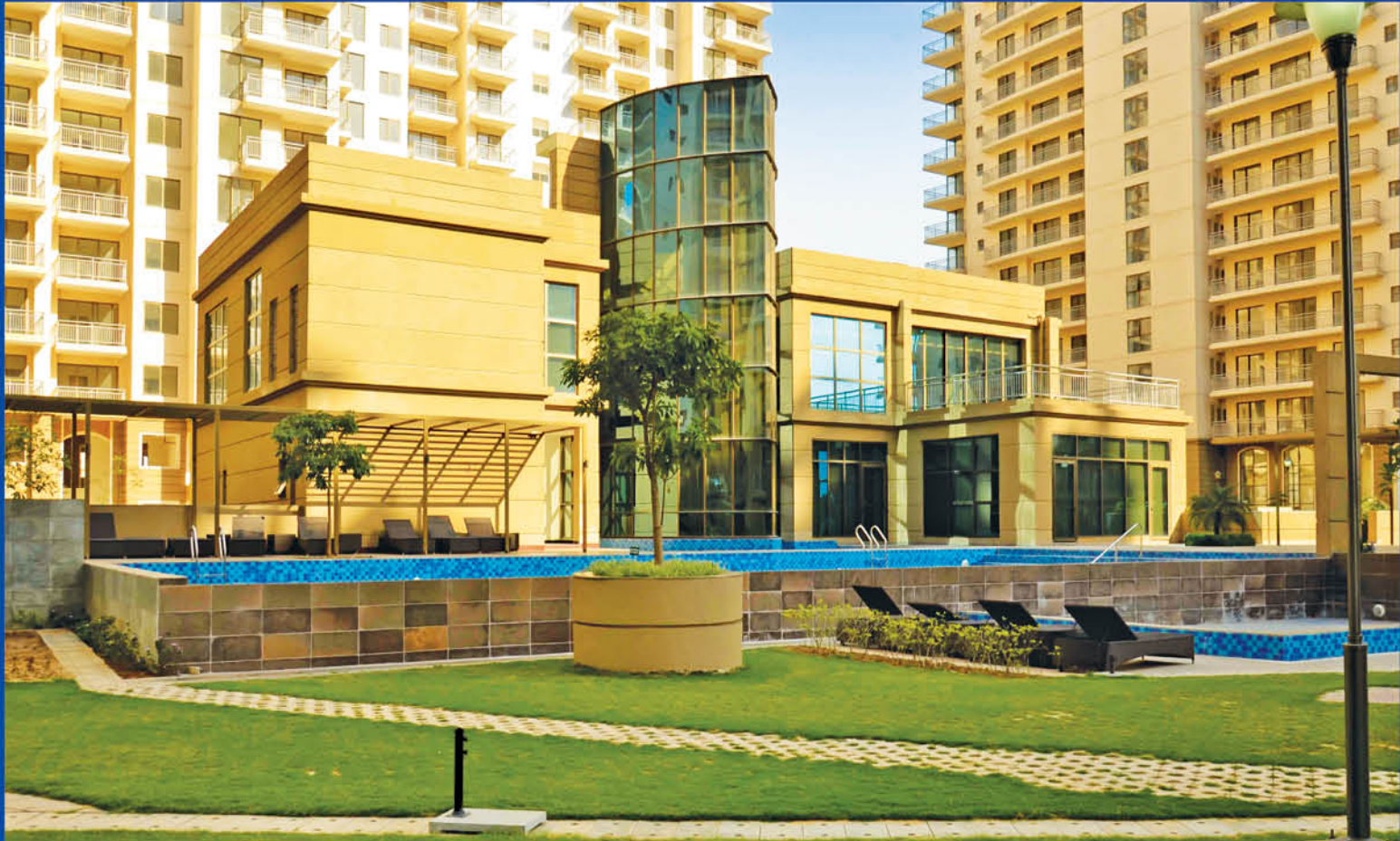
Godrej Frontier, Gurgaon
